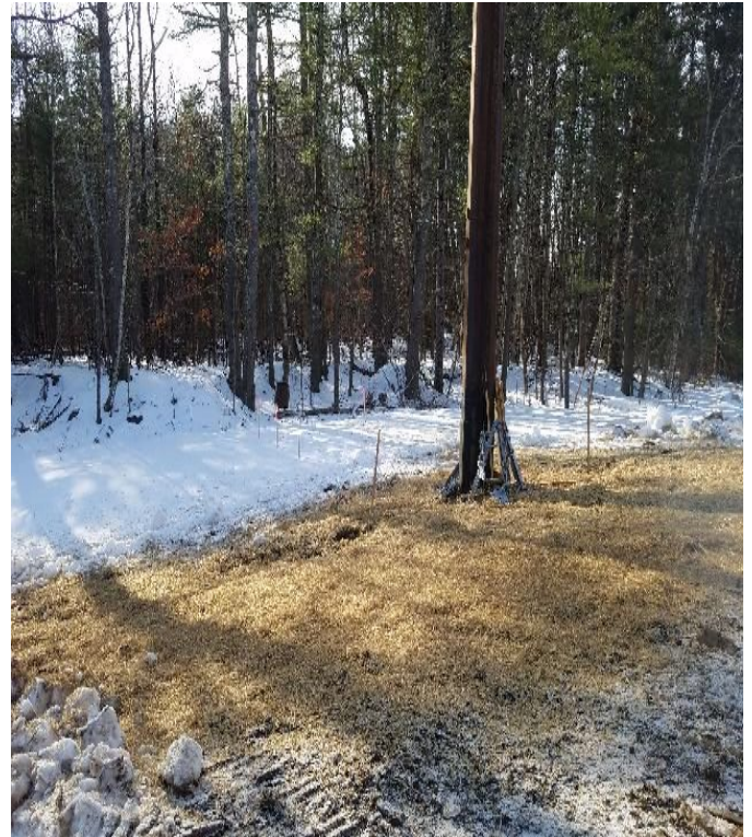
Fig 22: Str. 101 pole constructed. Viewing south. (01-08-20).
