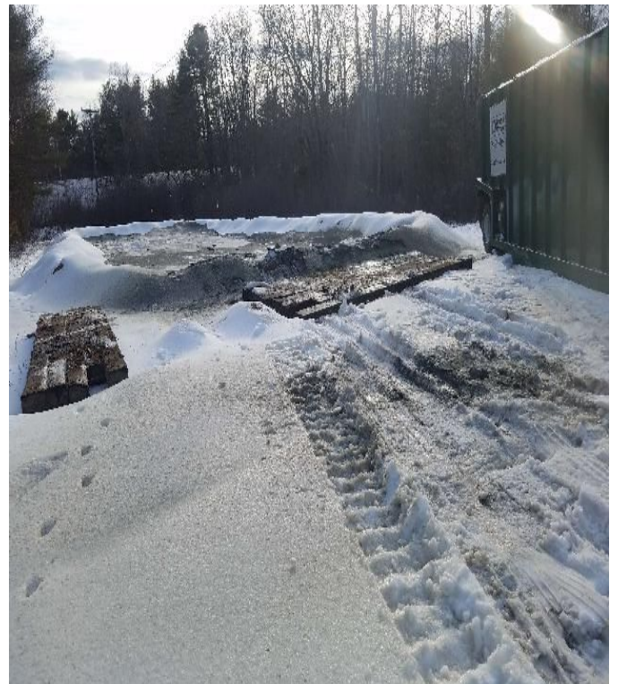
Fig 16: Dewater basin and frac tank for Str. 48 dewatering. Viewing southwest. (01-07-20).
