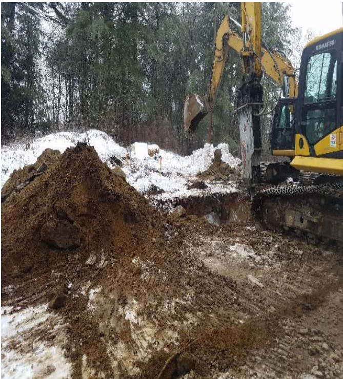
Fig 3: Crew hammering ledge for foundation at Str. 56. Viewing south. (01-02-20).
