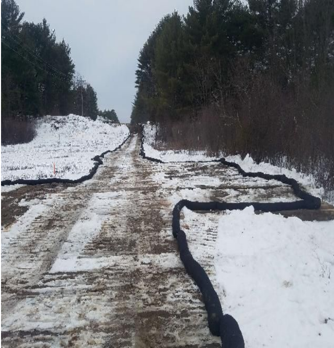
Fig 5: Crew installing filter sock along access through wetland DW31. Viewing west. (01-02-20).
