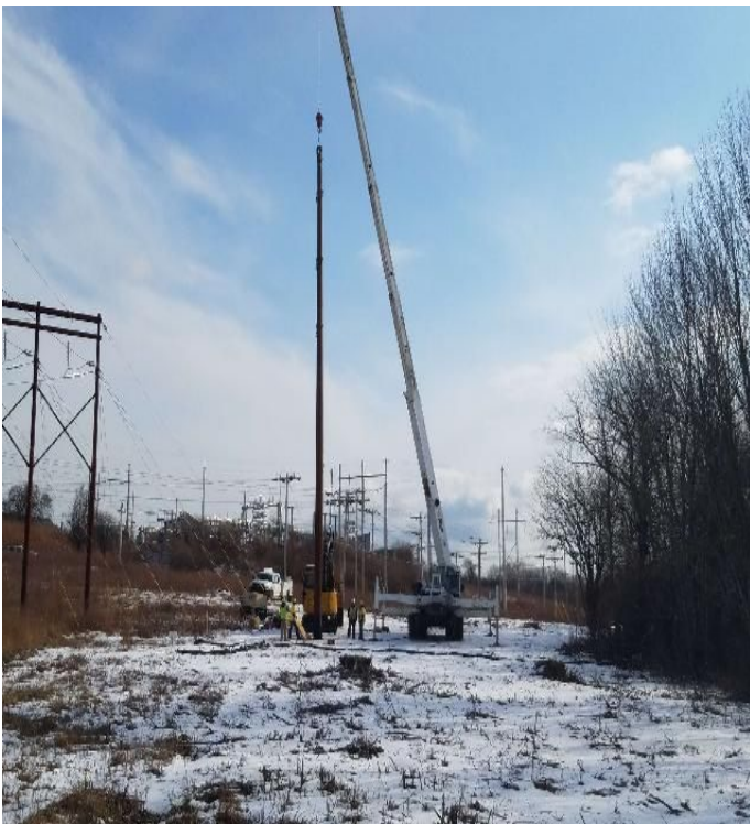
Fig 23: Crew standing pole for Str. 142. Viewing east. (01-08-20).
