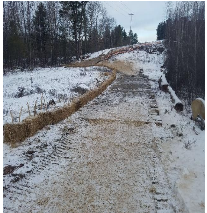
Fig 10: BMPs installed along access road between Strs. 47-46. Viewing north. (01-06-20).
