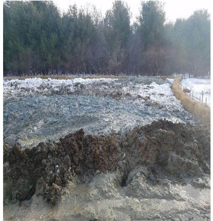
Fig 18: Soil from drilling Str. 48 foundations being used to build turtle nesting area. Viewing south. (1-08-20).
