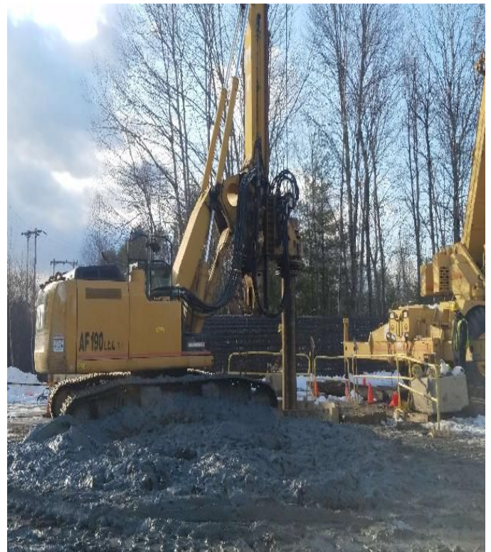
Fig 20: Drilling foundations for Str. 48. Viewing west. (01-08-20).
