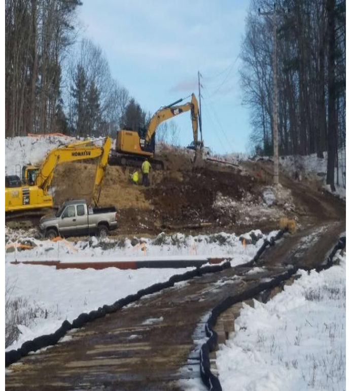
Fig 14: Crew setting foundation cans for Str. 57. Viewing northeast. (01-07-20).
