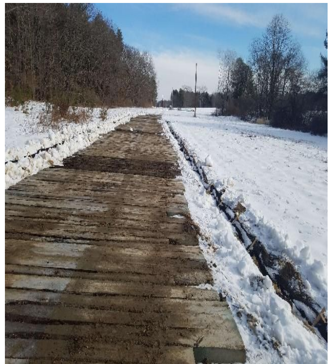
Fig 12: Filter sock installed along access road through wetland NW 10. Viewing northwest (01-06-20).
