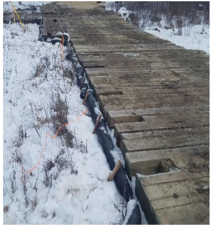
Fig 8: BMPs installed along access road through wetland DW56. Viewing north (01-06-20).
